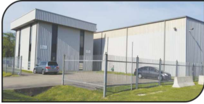
Distribution Center, Houston, USA
